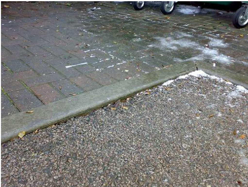
Figure 5. Threshold at Sainsbury's Huntingdon
